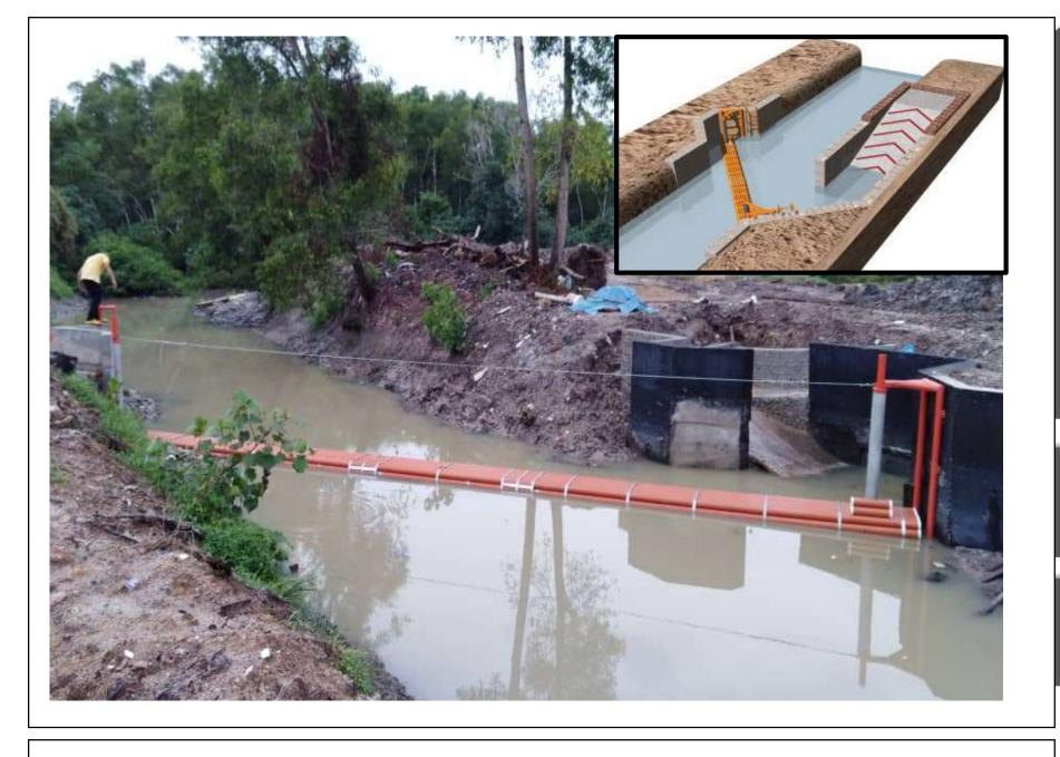
The MFRT is installed alongside a buffer that has a ramp for ground-strewn drainage.
