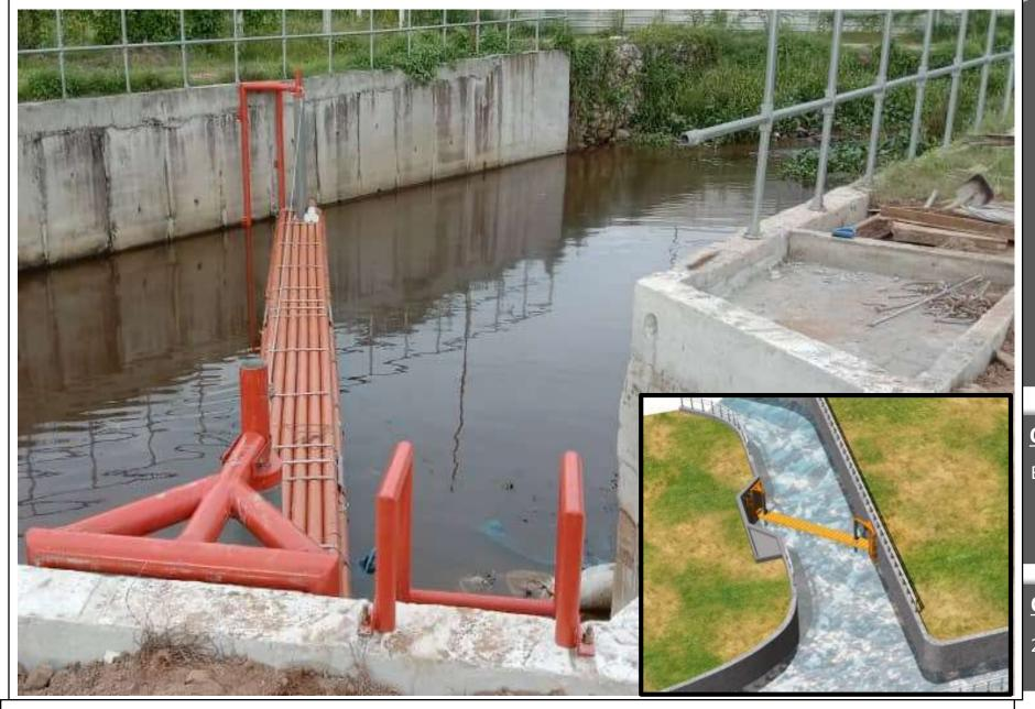
The 14 mtr-long MFRT is installed in a large trench along with 'sump' and garbage collection points.
