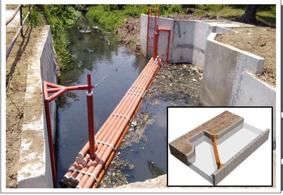
The MFRT was completed installed with sump in the trenches of The Garden of Peace. Pictures show The garbage collected in the sump room.
